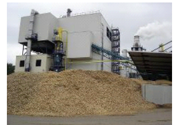
Woodchips and sander dust is ideal for a spreader stoker
