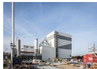
La construction de Tilbury Green Power.
