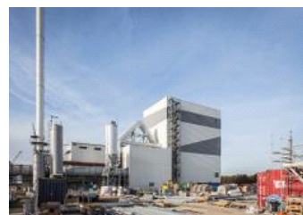
Le construction de Tilbury Green Power.
